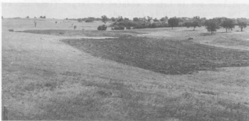
After installing drop inlet structure for grade control, and shaping
