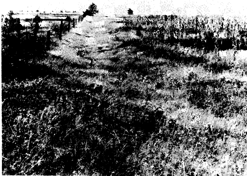
Figure 10-2 Same gully treated by filling, shaping and planting to grass
