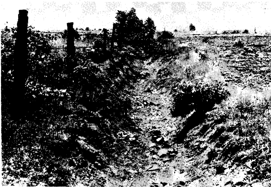
Gully caused by emptying terraces into an unprotected outlet
