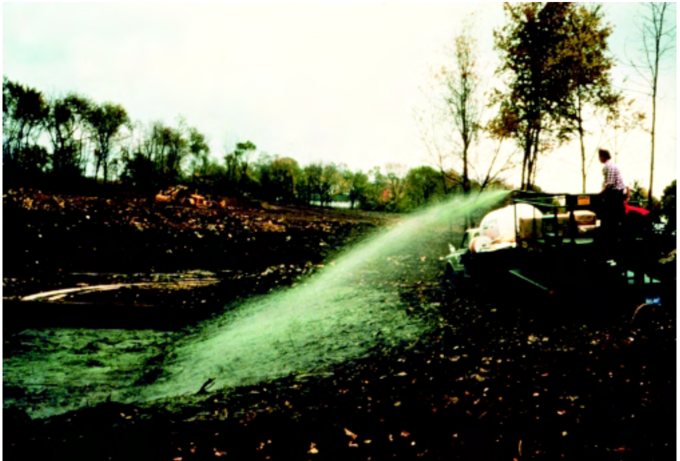
Figure 14–19 Seeding newly constructed drain
