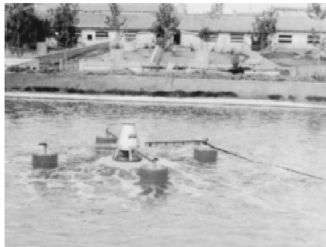
Figure 12-54 Floating aerators for liquid waste aeration (courtesy Aeromix Systems Inc. and AgriBusiness International, Inc.)
