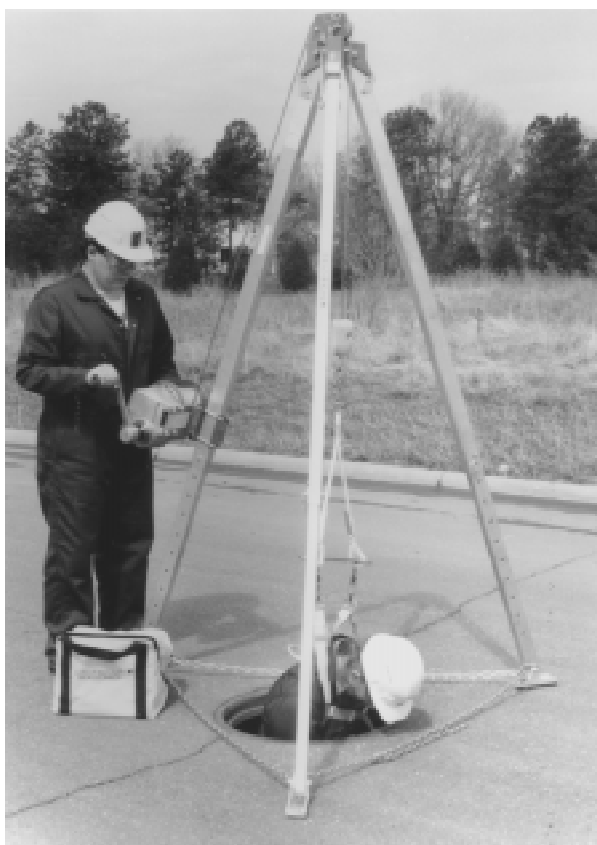
Figure 12–117 Tripod, winch, and harness (courtesy D B Industries, Inc.)
