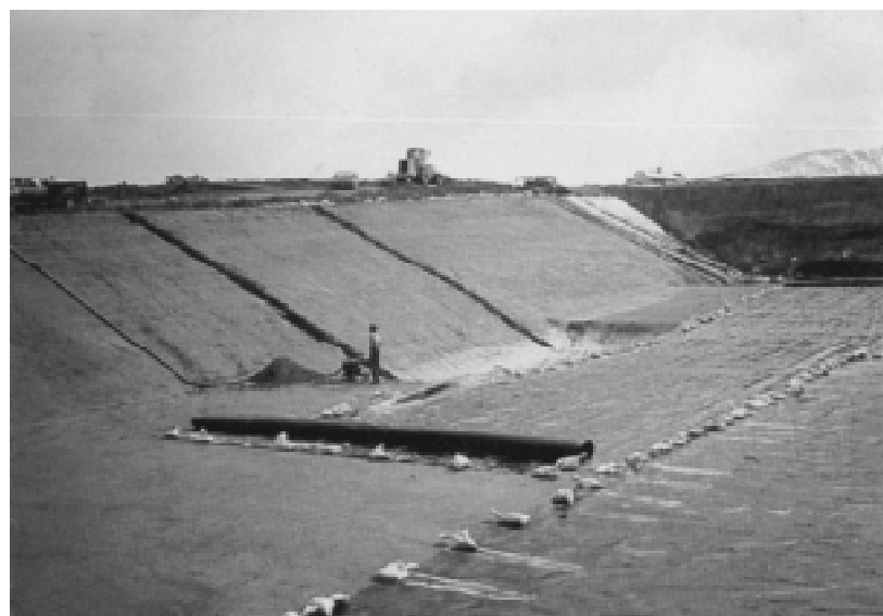
Figure 12-38 Membrane liner installation for earthen basin (courtesy Hoechst Celanese Corp.)
