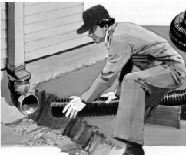
Figure 12-7 Corrugated plastic drainpipe (courtesy Advanced Drainage Systems)
