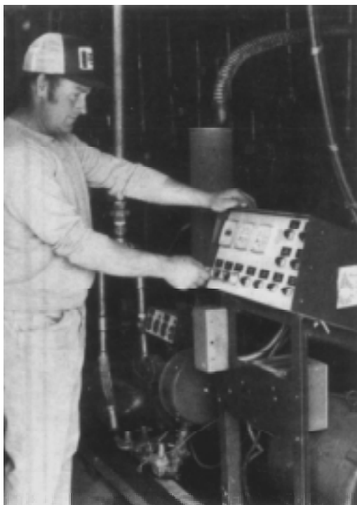
Figure 12–105 Biogas production equipment
