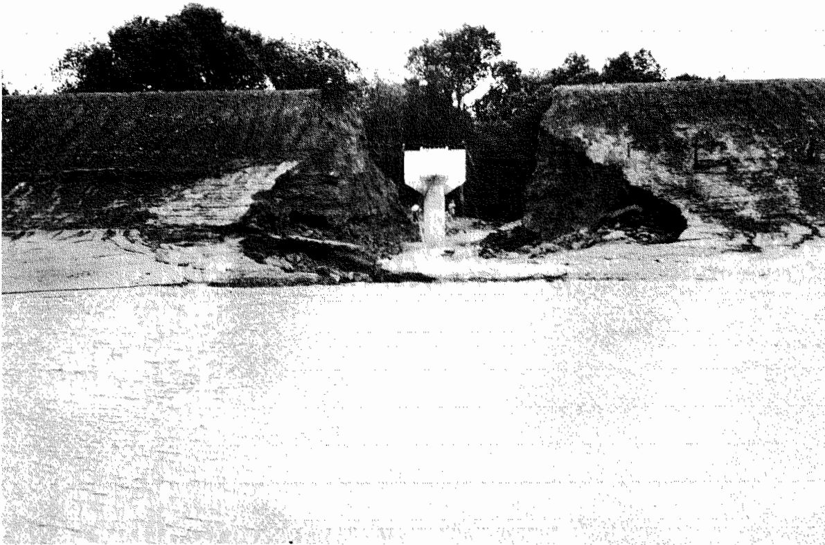
Figure 7. Failed Embankment Constructed of Dispersive Clays.
