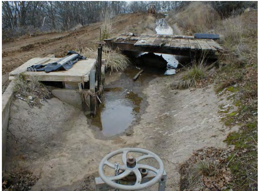
Photograph 2. View is looking upstream in the Talent Canal at the Crooked River Siphon entrance. The StarFlow instrument was installed upstream of the wooden bridge. This section of canal experiences backwater when the spill to the river is not operated. The canal capacity is about 15 cfs.
