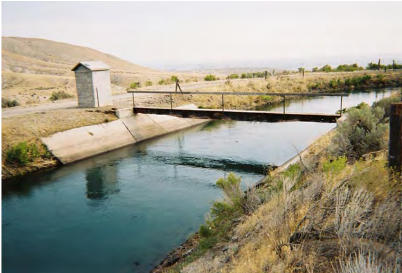
Photograph 6. At the South Canal site, flow depths varied from 3.5 feet to 5.5 feet during the 2003 irrigation season. Current meter measurements were made from the foot bridge.
